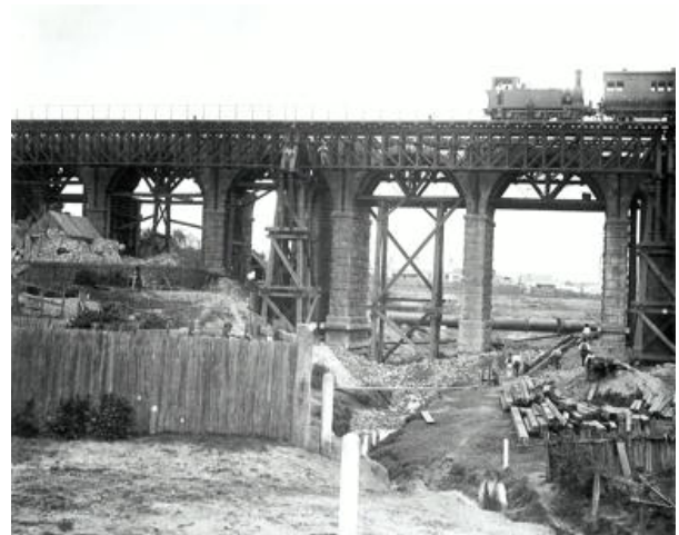
Railway bridges, Lewisham (1887)
